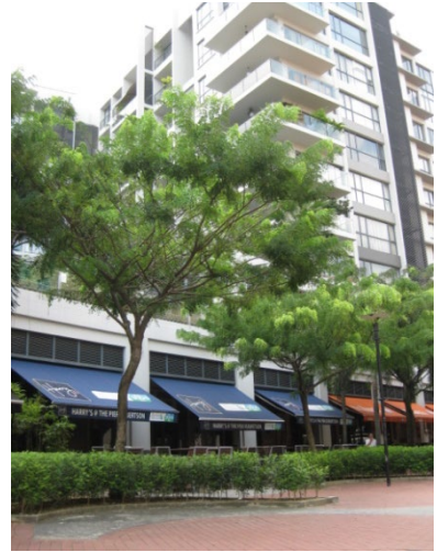
Figure 3-1: Awnings are to complement the scale and rhythm of the development façade, e.g. correspond to the column locations. Applicants should also seek clearances from SCDF on the location and extent of protrusion from the building façades.
