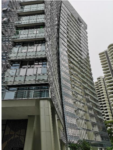
Curved façade walls
