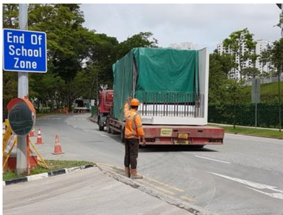
Traffic controller guiding delivery trailer
