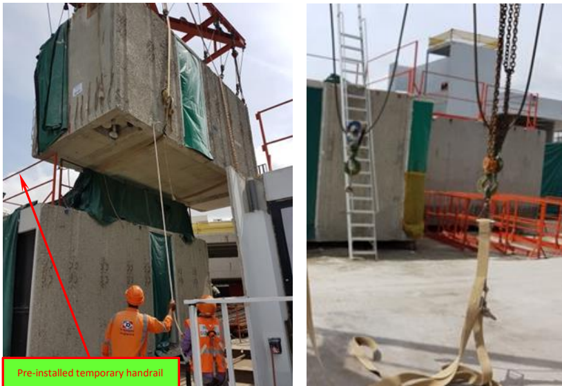
PPVC units with pre-installed temporary handrails
