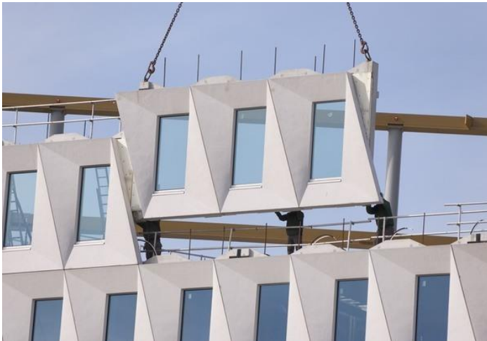
Façade panel which is fixed into position from building interior
