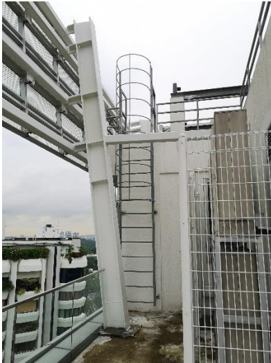
Cat ladder located at edge of roof
