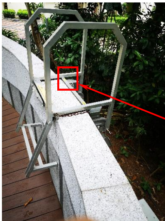
Foldable landing with safety pin for locking into position
