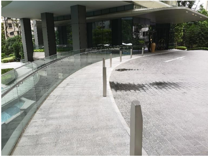
Bollards provided along edge of driveway
