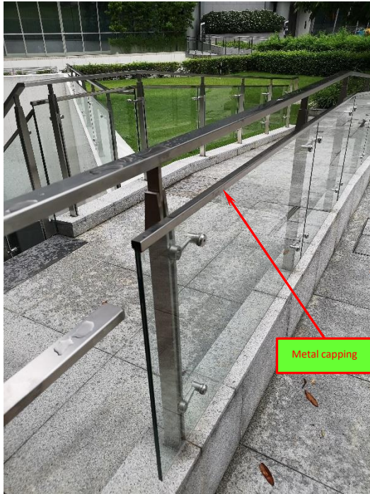
Balustrade with glass panels
