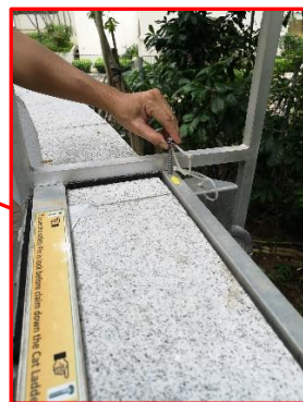
Foldable landing with safety pin for locking into position
