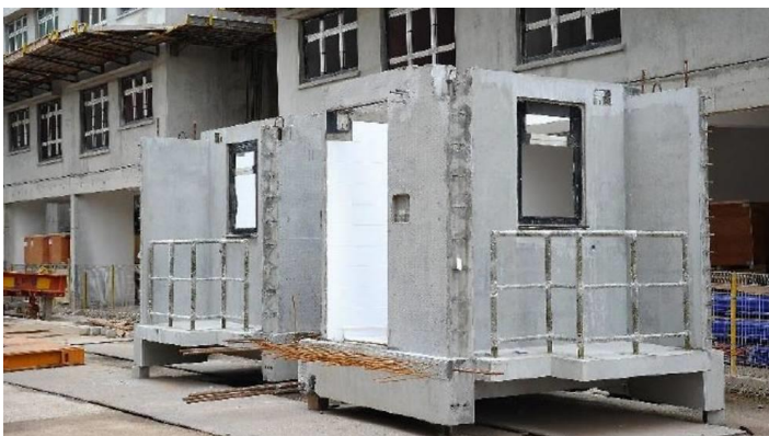
Railing installed before entire precast unit is lifted up
