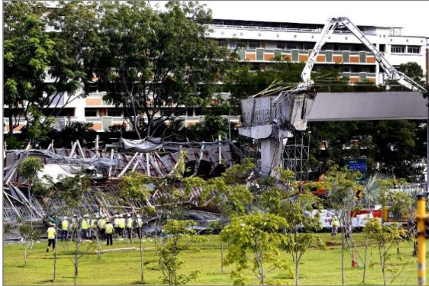
Collapse of bridge under construction during concrete pour
