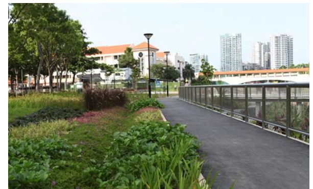
Bioretention Swale at Kallang River Potong Pasir
